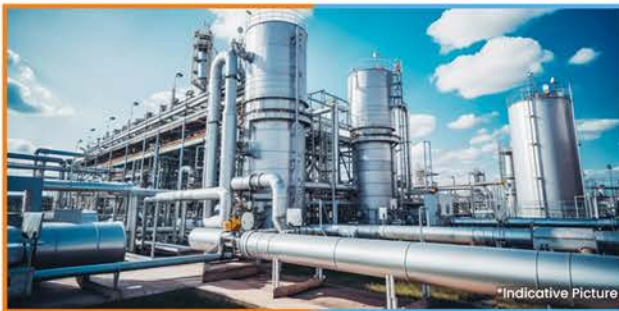
2200 TPD Chlor - Alkali Plant, India
