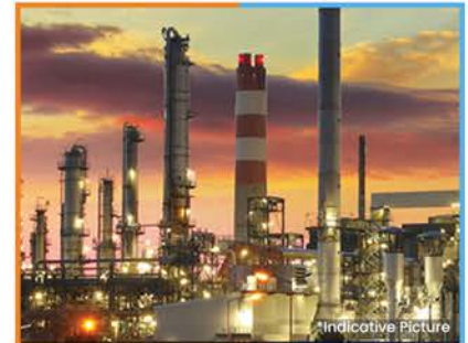
Propylene Purification Plant, India
