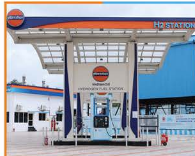
Hydrogen Fueling Station, India
