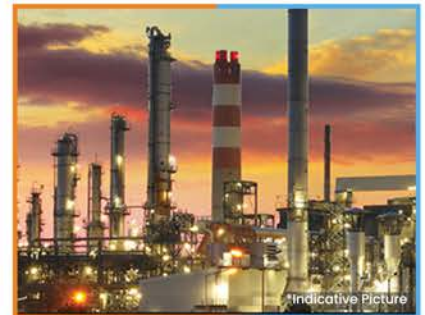
Propylene Purification Plant, India
