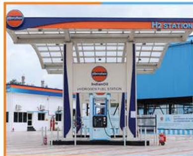
Hydrogen Fueling Station, India
